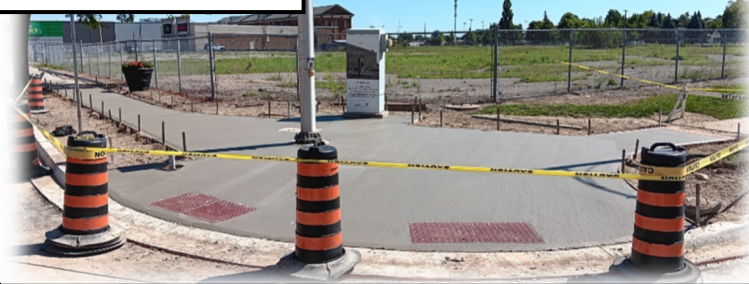
New Concrete sidewalk and ramp at Ross and Talbot
